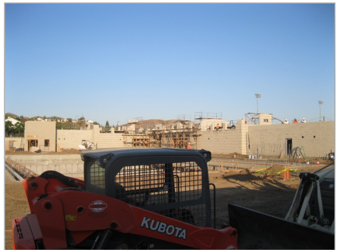
2. Building Masonry 80% complete
