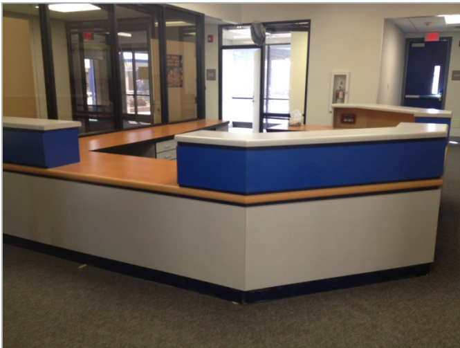
1. Completed reception desk, countertops, fire alarm annunciator panel, data, and light fixtures at the Main Office.-Phase Nine
