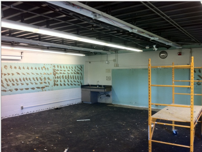
1. Demolition and removal in new computer lab. -Phase 1A
