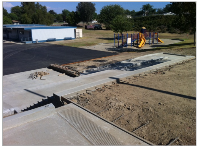
2. Switchback ramp and stairs from the upper field to lower field.
