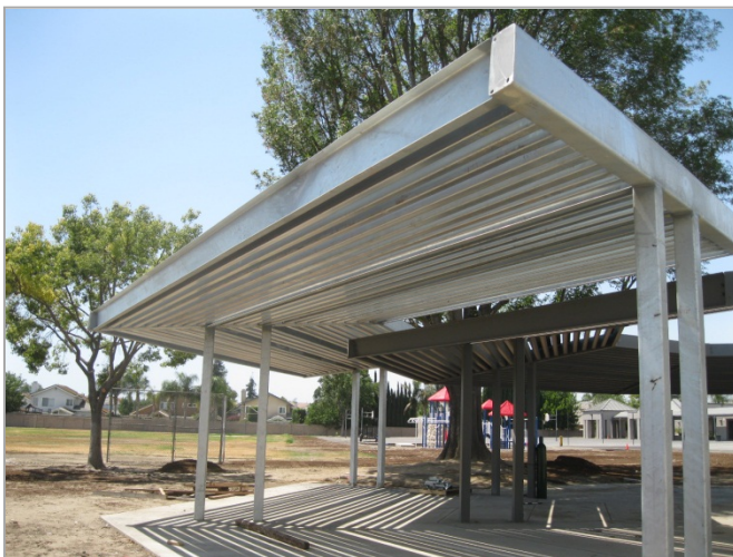
3. Shade shelter steel installed.
