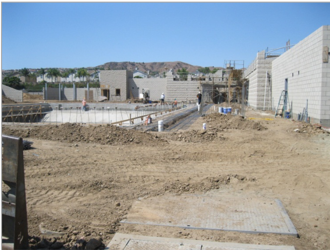
1. Pool Shotcrete/Concrete done. Gutter Drains In Progress
