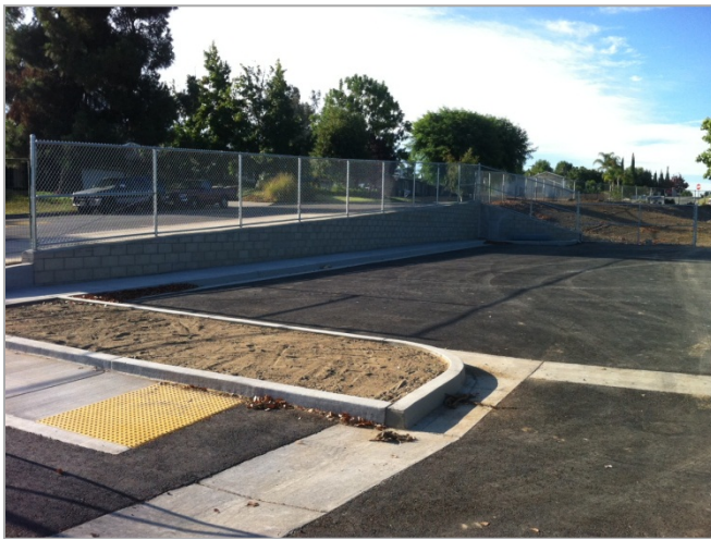
1. Trash enclosure and front parking lot nearly complete.
