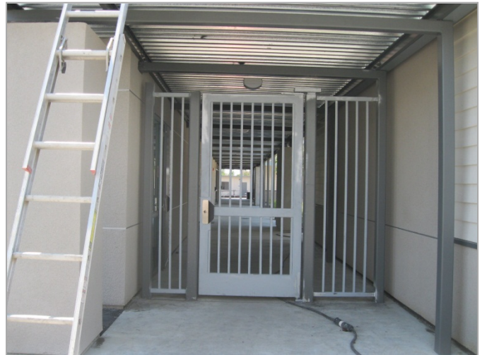
2. Fencing and gates installed.
