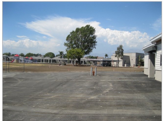
4. Playground grading and soil amendments.
