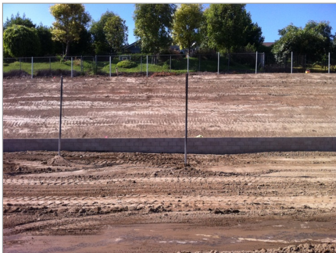
3. Slope ready for irrigation and planting.
