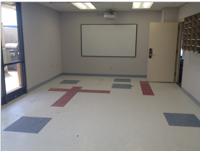
3. New vinyl composite tile, light fixtures, ceiling tile, and interactive whiteboard and projector at the Teachers Lounge.-Phase Nine
