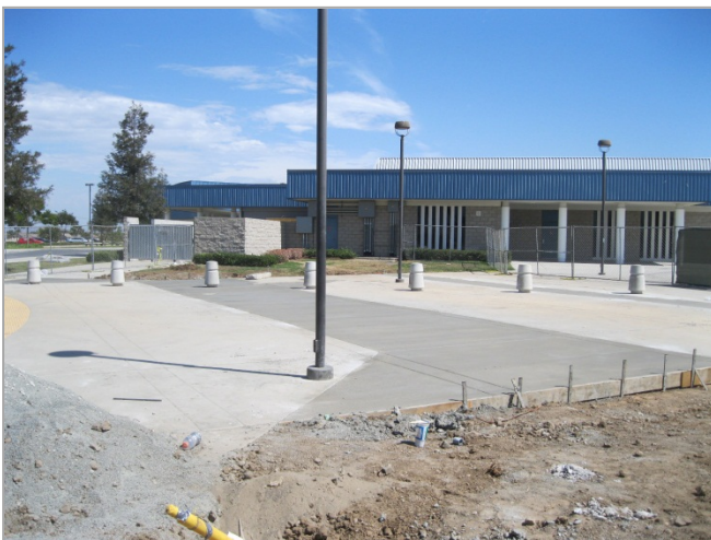
3. Cross-campus tie-in trenching complete and repaved
