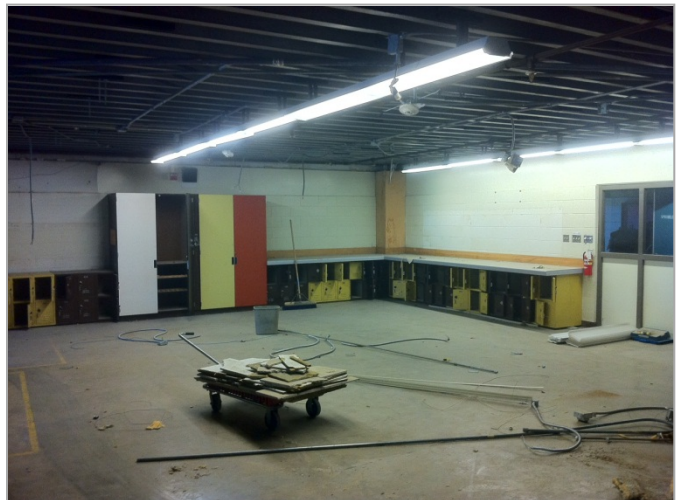
4. Demolition and removal in new library. -Phase 1A
