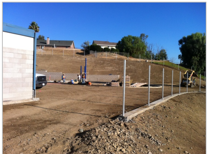
4. Playground equipment installation in progress.
