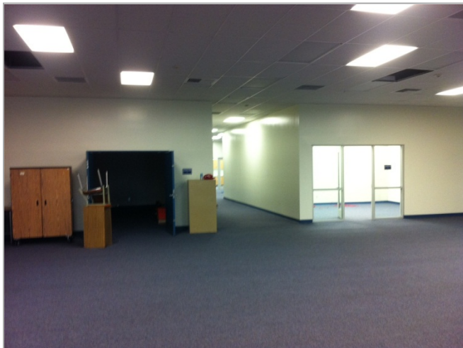
3. New offices and storage rooms in progress.
