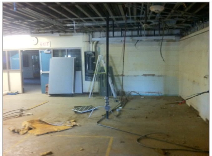
2. Demolition and removal in new library. -Phase 1A
