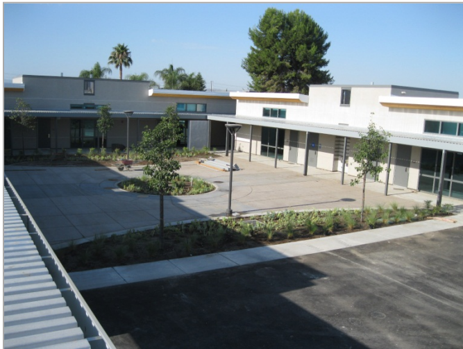
1. Courtyard hardscape complete.
