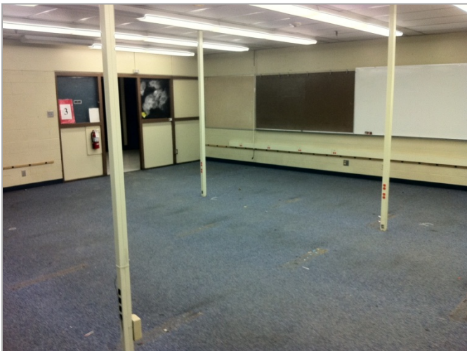
3. Demolition and removal in special education classroom. -Phase 1A
