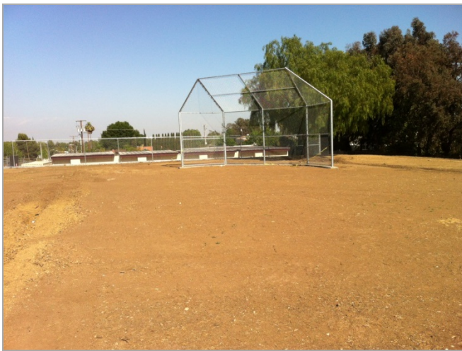
1. Backstop installed at new field.
