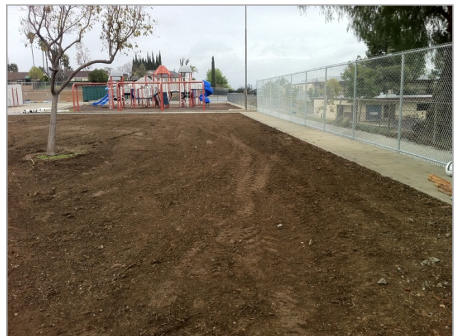
4. New walkway to playground equipment complete.
