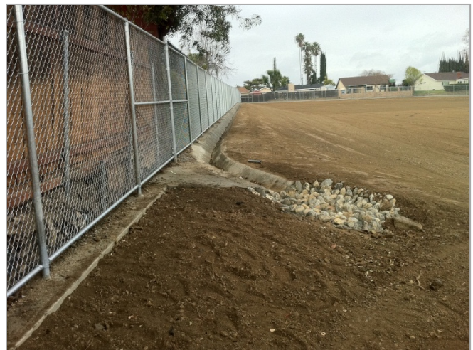
2. West property line complete and ready for hydroseed
