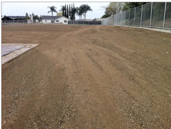
3. North slope complete and ready for hydroseed.
