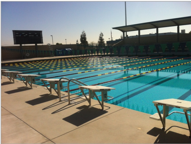
1. Pool is ready and in use.
