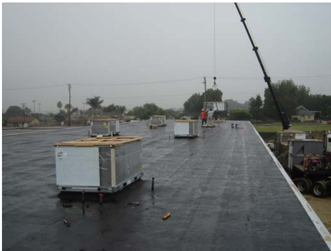
1. Installation of rooftop a/c units.
