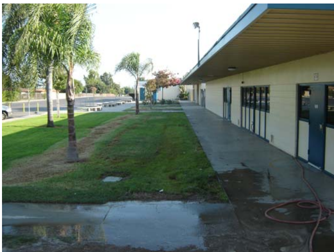
3. Completed sitework in front of campus.
