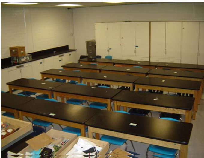
3. New flooring and paint in classroom. Furniture placed back into classrooms.
