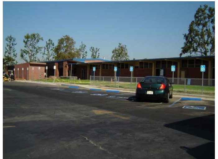
2. New ADA parking in front of school. New Restroom building (left).
