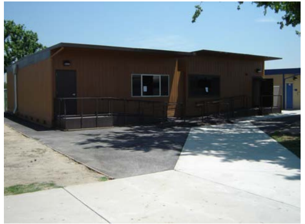
2. Completed Interim Housing units.
