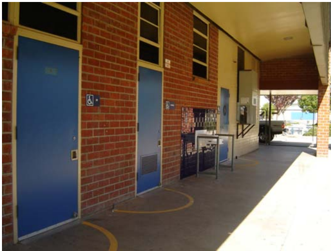
1. New ADA signs and drinking fountain and tile.
