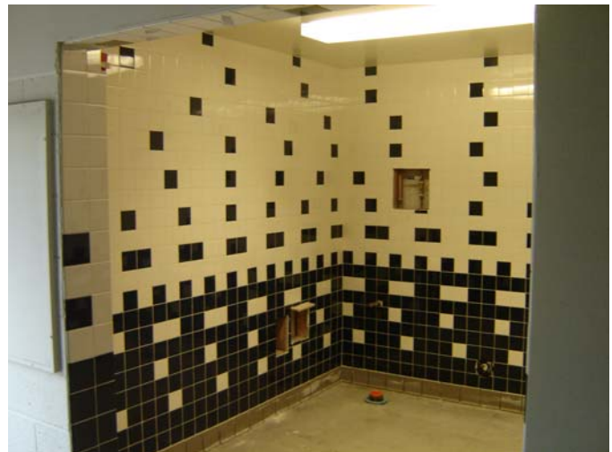
4. Ceramic tile at Girls' Restroom in Locker Room.
