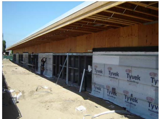
2. Installation of exterior wall moisture barrier.
