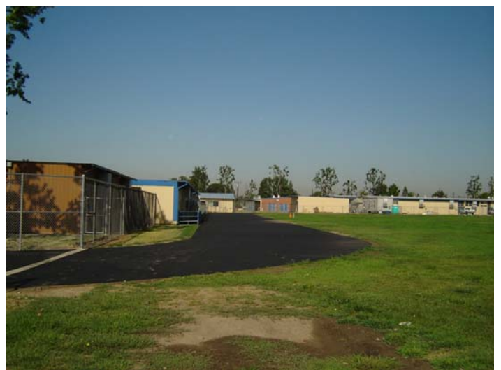
4. New Fire Lane.
