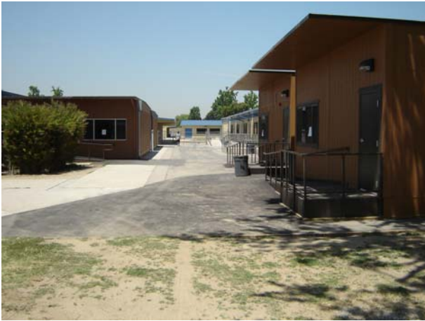
1. Completed Interim Housing units
