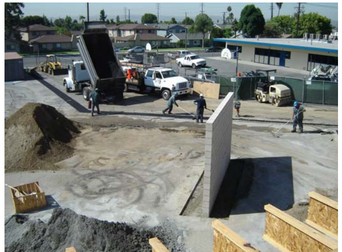
2. Completed concrete stemwall footings.
