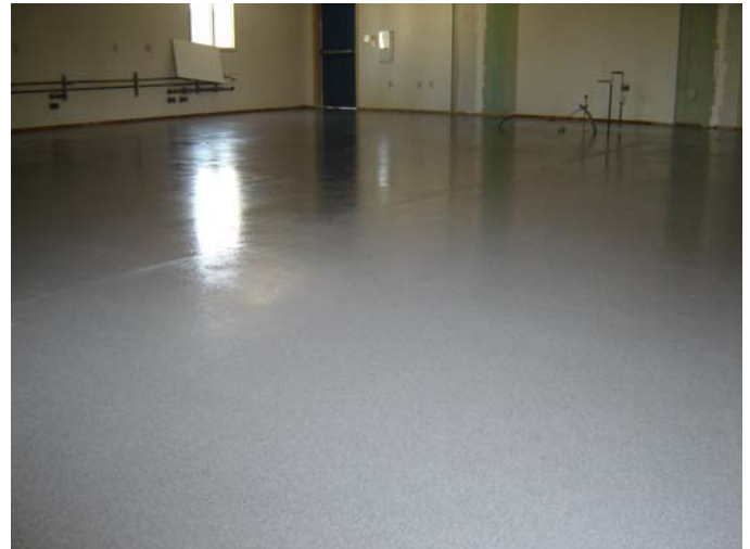
2. New epoxy flooring in Relocatable Classroom.
