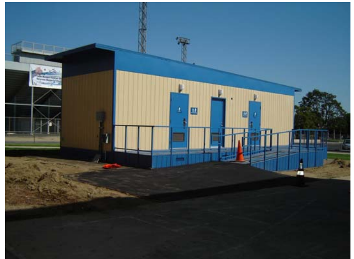
4. New Relocatable Restroom Building near gymnasium.
