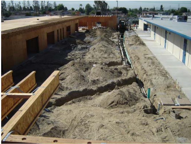
1. Vapor barrier over sand for concrete slab.
