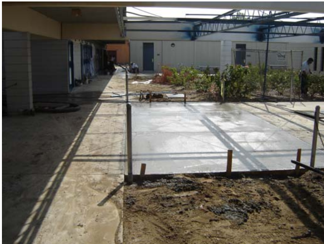
3. Conduits for electrical and low voltage systems.
